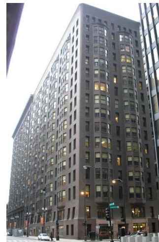
Monadnock Building, de Burnham e Root. Chicago, 1891 Fonte: wikipedia.org
